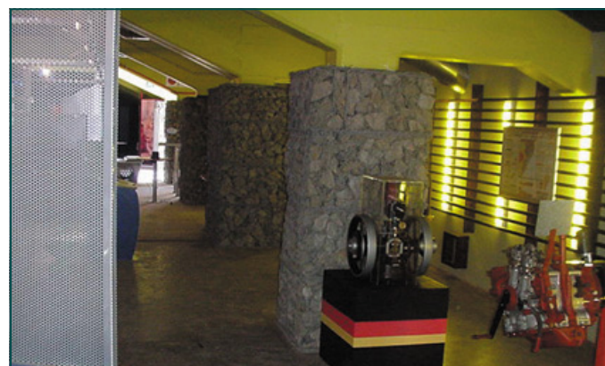
Gabion cladded columns
