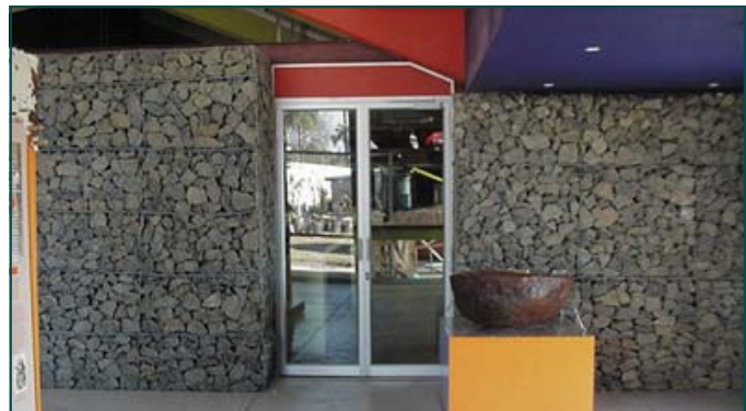
Cladded Gabion Walls
