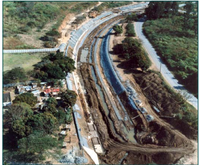
Aerial view of Booth Road canal during construction
