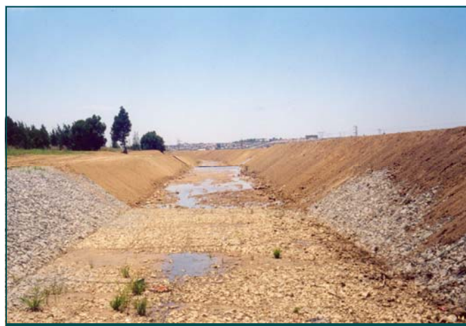
Channel lining immediately after installation
