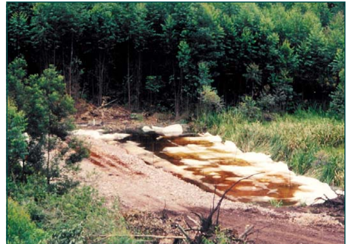
Laying the FlexMesh™
