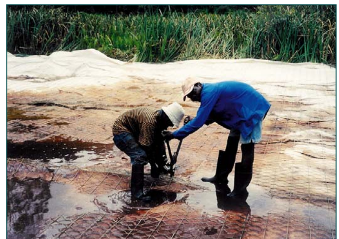
Lacing & pegging down FlexMesh™
