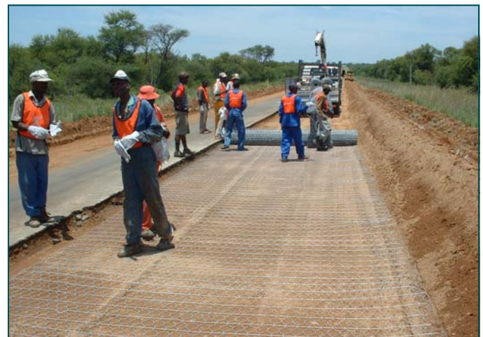
Unrolling the mesh manually
