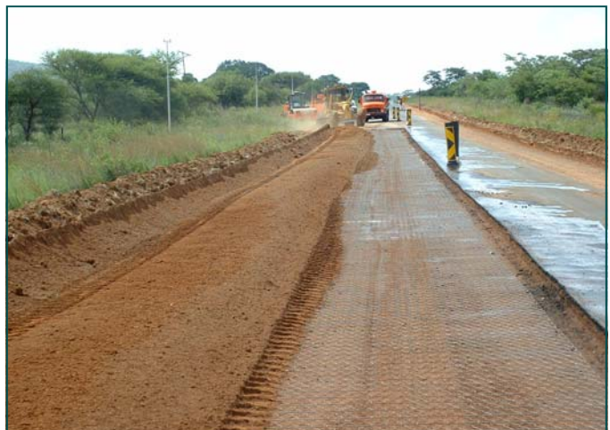
Placement of second layer Date: Jan 2003
