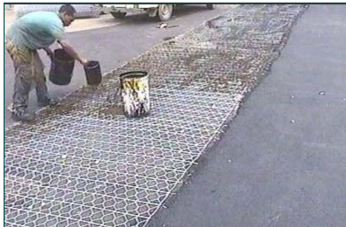
Application of tack-coat
