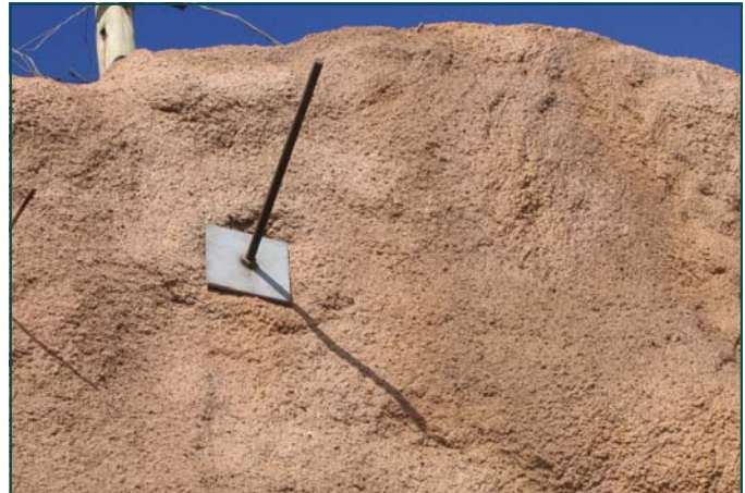
Installed Soil Nail Date: Mar 2005
