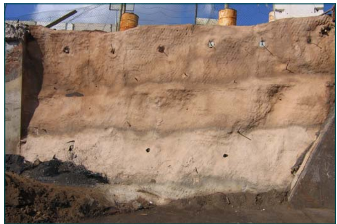
Finished soil-nailed and shotcreted face Date: Mar 2005
