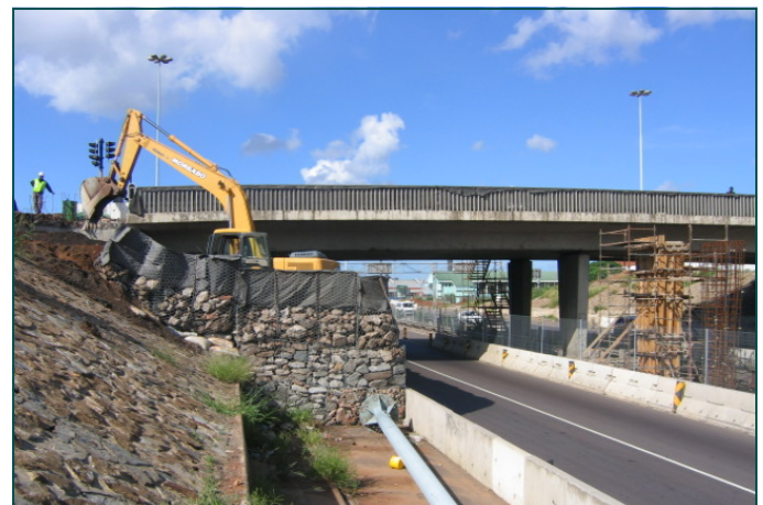
Temporary Gabion Wall
