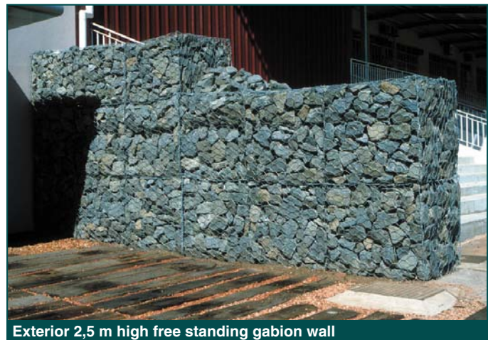
Exterior 2,5 m high free standing gabion wall
