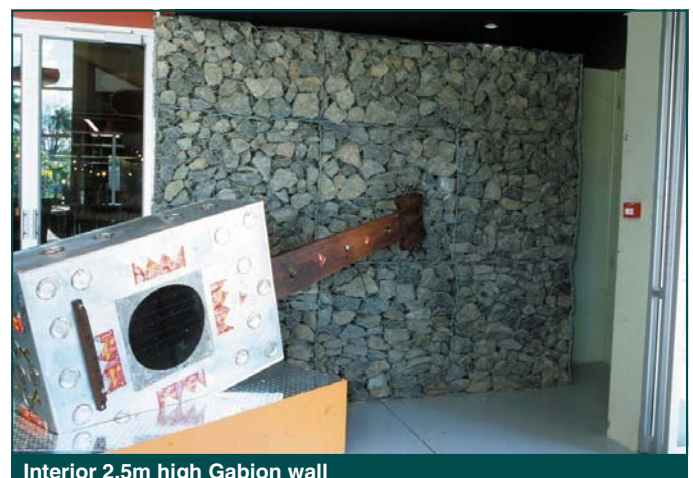
Interior 2,5m high Gabion wall
