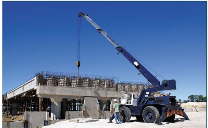
Diep Rivier bridge with crane installing MacForce panel
