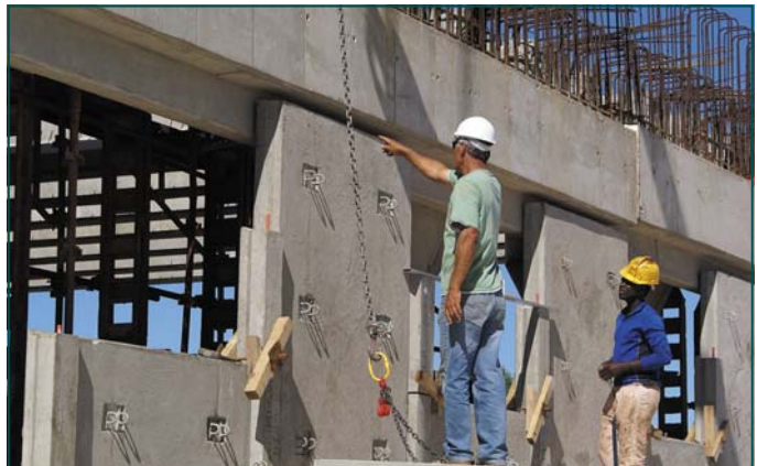
Checking clearance between MacForce panel and bridge
