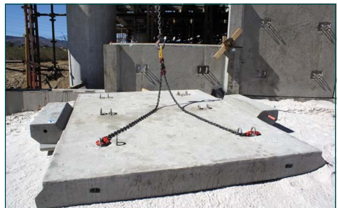
Special Panel ready for placement
