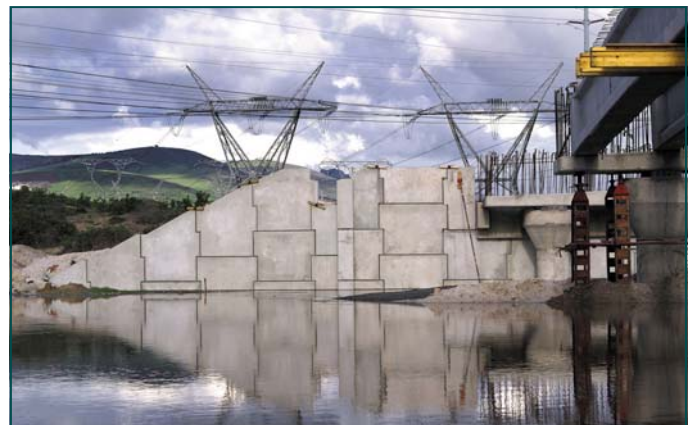
A calm flow past the Diep Rivier bridge, MacForce abutment
