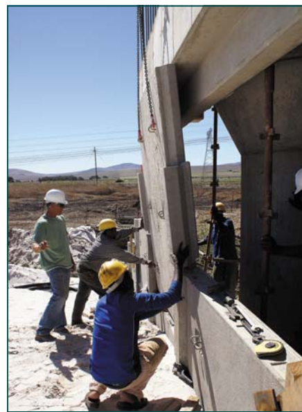
Careful adjustment for placing panel under bridge soggit
